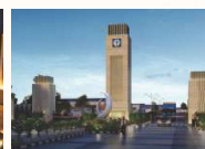
MANGLAM INDUSTRIAL PARK - II
